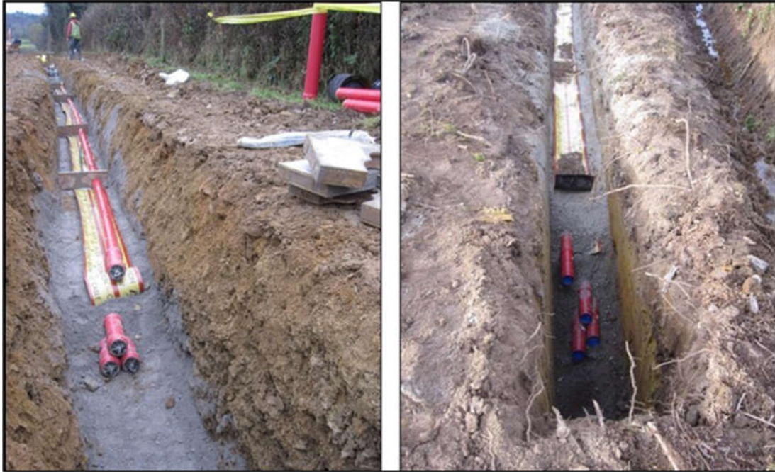
Plate 4-7 Standard Cable Trench View
