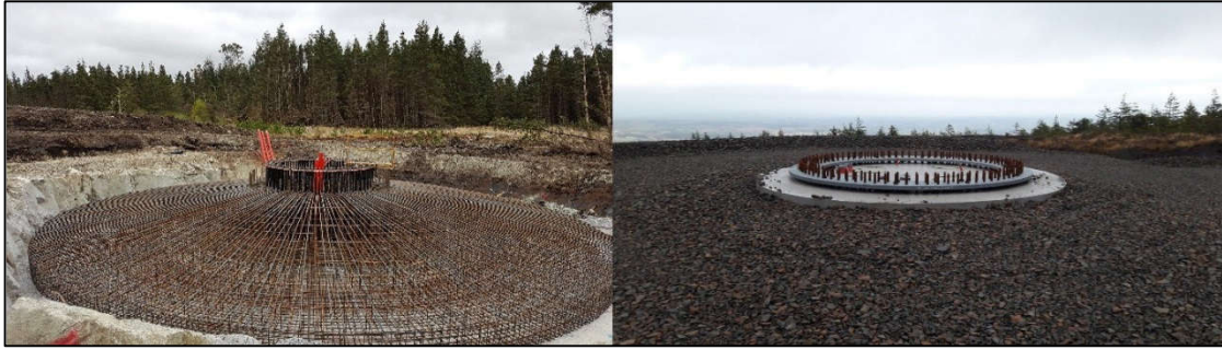
Plate 4-2 Turbine 'Anchor Cage' and finished turbine base
