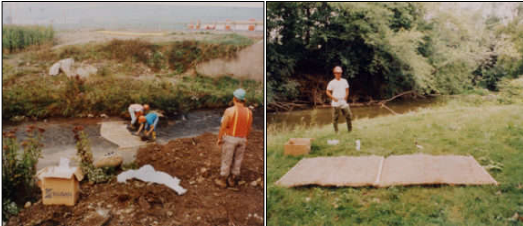
Plate 4-5 Typical Sedimat Details (Source: https://www.hy-tex.co.uk/ )
