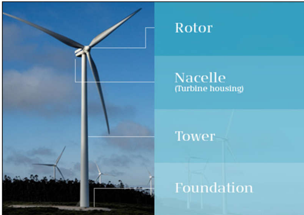
Plate 4-1 Wind turbine components
