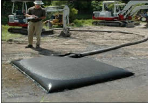
Plate 4-3 Silt Bag with water being pumped through
