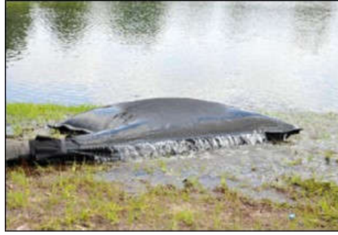
Plate 4-4 Silt bag under inspection
