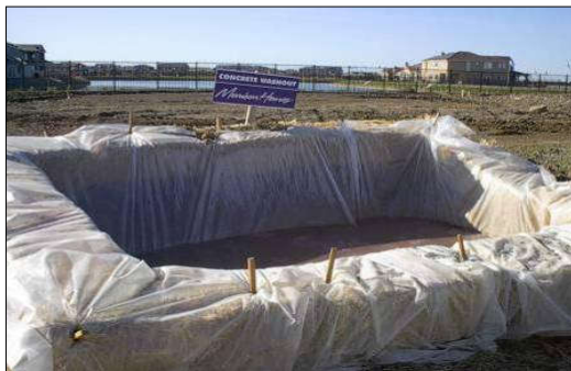
Plate 4-3 Concrete washout area
