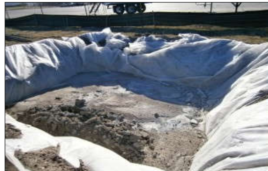
Plate 4-4 Concrete washout area
