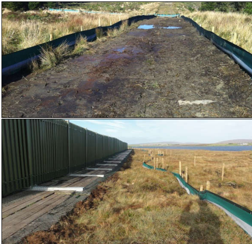
Plate 4-6 Silt Fence Details
